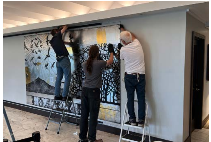
Installation of the “Deep Mystery” mural.
